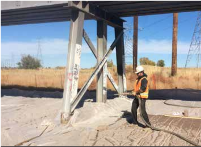
Prepping heavy steel with 20/40 garnet blasting media, this Painters USA crew member minimizes dust and achieves the ideal surface profile.
