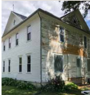
Brian Denlinger used a Diamabrush Wood, Decks, and Siding Tool to remove decades’ worth of paint from this historic home, restoring it to its original beauty.
